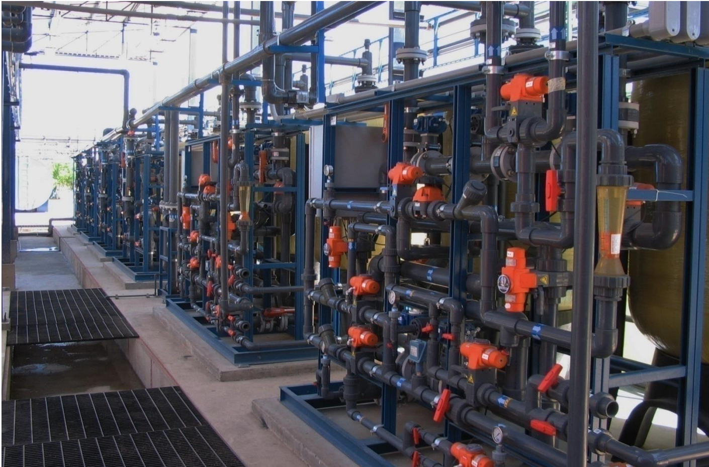
Duplex 175 GPM IX System with carbon and media filters
